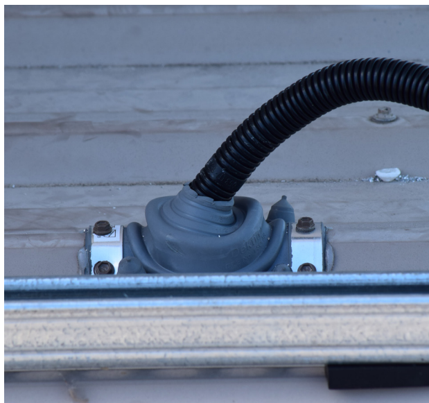
Figure 17: A Dektite* with a metal roof flashing
